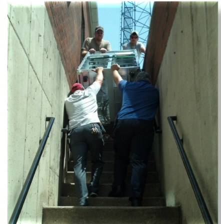
Pictured: Telecom's Geezer and Paul Bernard helping Chapel Electric bring in a battery cabinet for the generator room.
